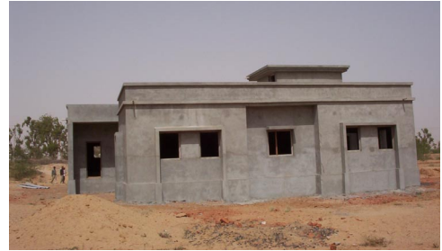
Rear view (looking east).
