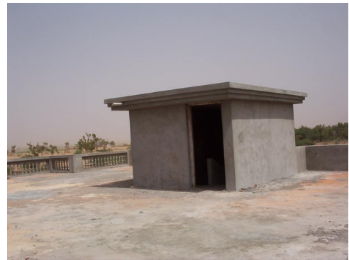
Rooftop and stairwell.
